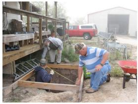
cementing and wired rebar to it. The final part was to get it perfectly level and put support boards in prep for the cement pouring. The idea, of course, is to keep the perfectly level base from being dislodged during the cement pouring. The cement cannot be delivered on a weekend so Charles and I will have to make sure there are no voids in the concrete and smooth out the top. I will have a report on that hopefully very soon.
